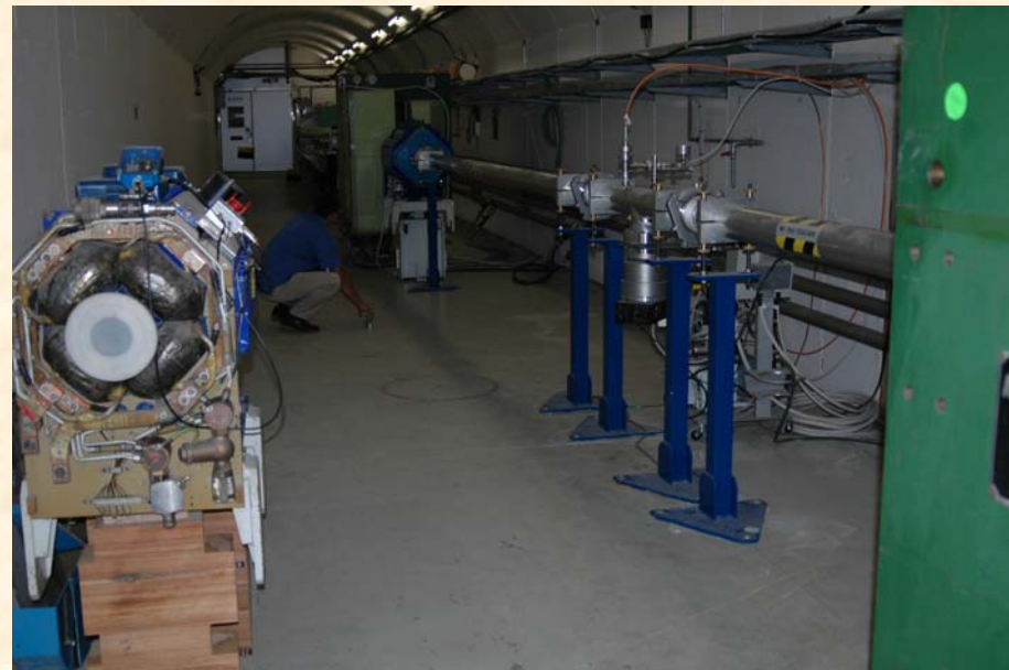
Tunnel Width 400cm (158")
