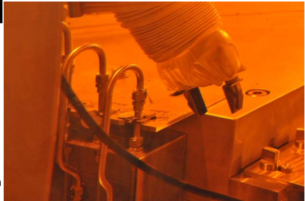
Re-connection of utilities between Target Cart and Facility
