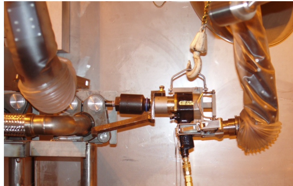
Torquing of Coolant Line Flange
