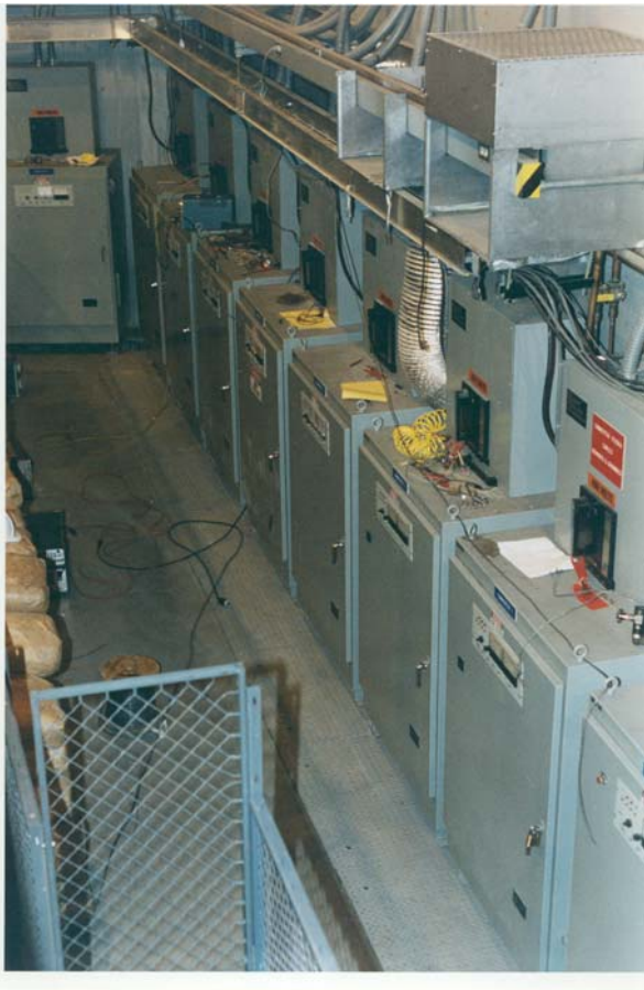
PTF Power Supplies
