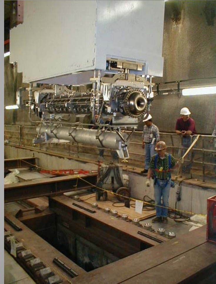
New NuMI Horn 1 and Beamline Positioning Module Chase Installation
