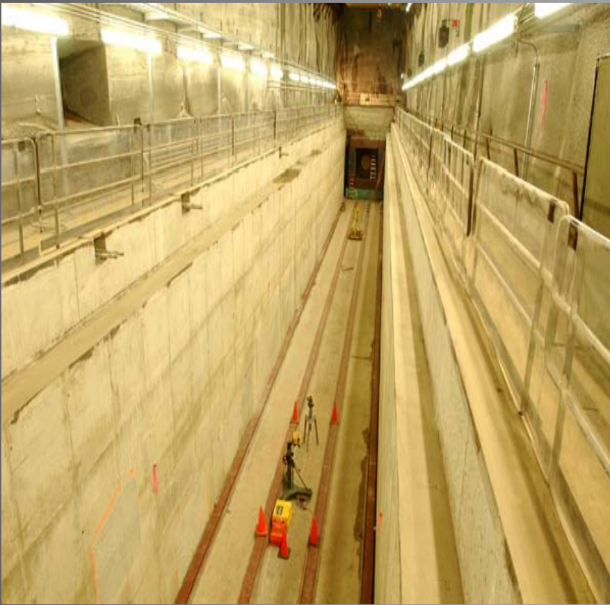
Concrete Lined Beamline Chase Walls and Base Provided by Civil Construction
