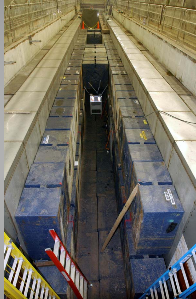
Beamline Chase Steel Constructed Using Duratek Steel Blocks
