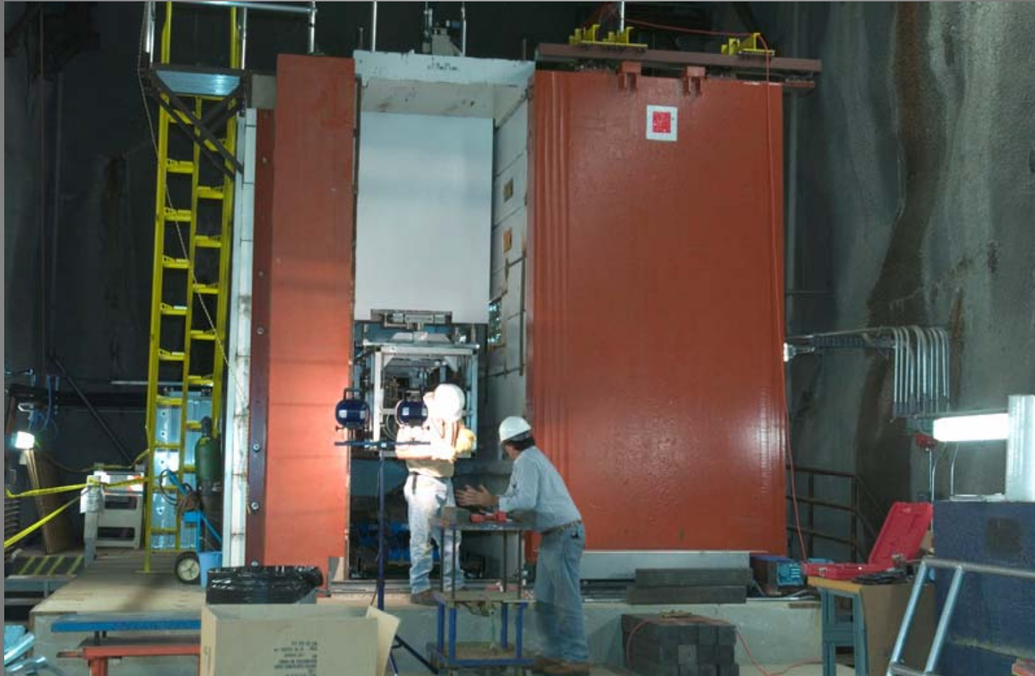
NuMI Workcell for Failed Component Replacement (Image shown is that of new components during installation)
