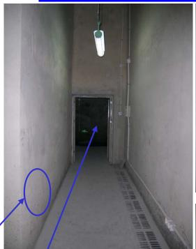
Door of gas mixing room, gas cylinders will be entering gas rooms through this door. The door is 1.2m wide and 2m height.
