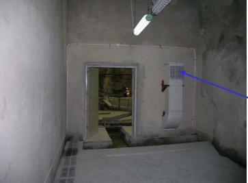
View from gas mixing room to EH#1, water pool can be seen through the door. The Air ventilation pipe is installed on the wall. Fresh air flows into the gas mixing room through this pipe. The air circulation is driven by this pipe and the exhaust pipe in the gas room, which is under negative air pressure.
