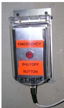
Fig. 14. Emergency shut off switch. To use the switch lift the cover and push the button.
