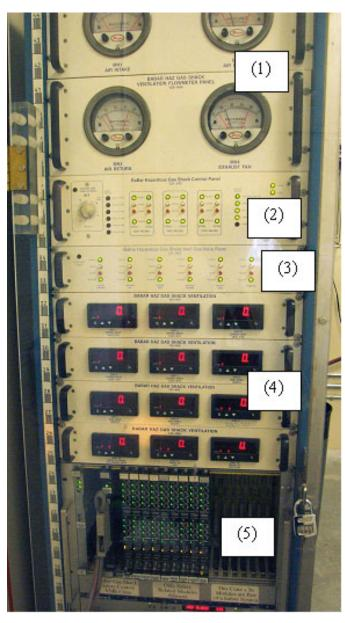
Gas Shack Control Panel: safety system independent of experimental control system.
